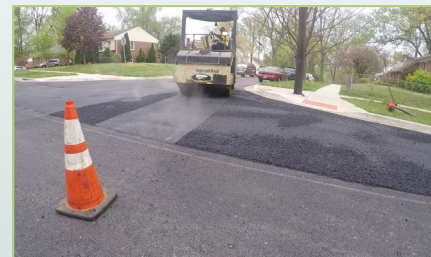
New asphalt is placed and compacted
